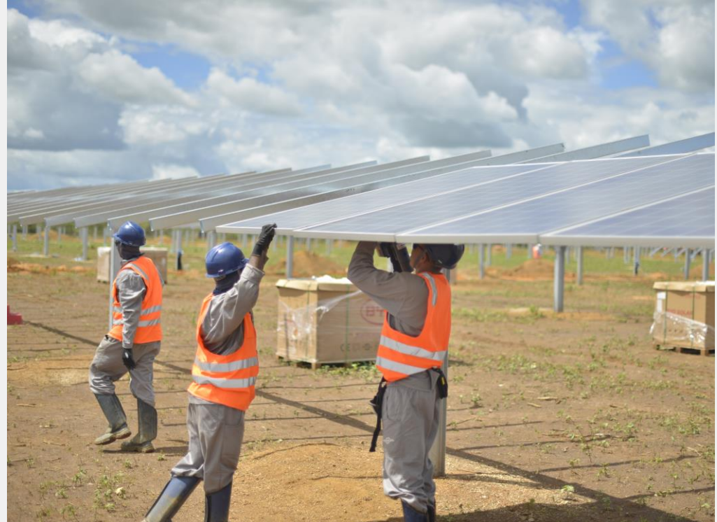
Module installation at the 162 MW Apodi site in Brazil
